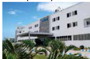
Rudrapur Plant (Green Building)
