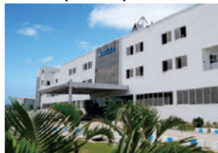
Rudrapur Plant (Green Building)
